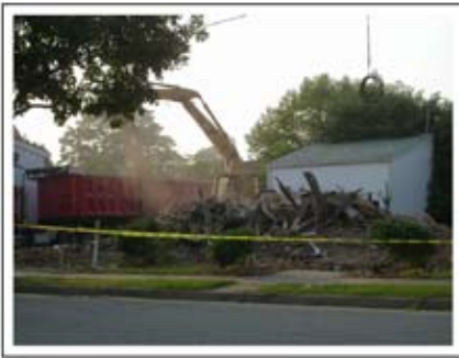
306 Wolfe St., Fredericksburg under demolition
